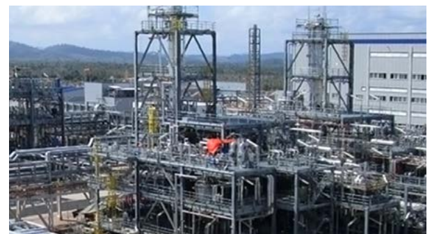
SOUTHEAST ASIA - H 2 S Production Facility, two trains each 60 MTPD. Licensed & Engineered by Unitel Technologies.
